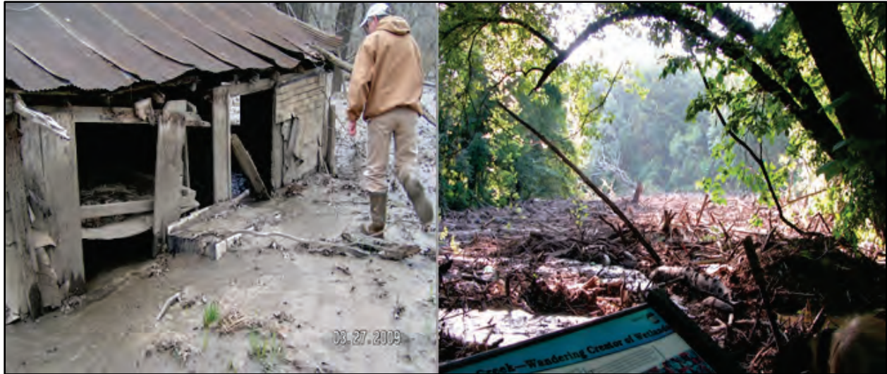
Figure 1-5. Excessive floodplain sediment deposition (left) and log jams (right) within Pershing State Park.
