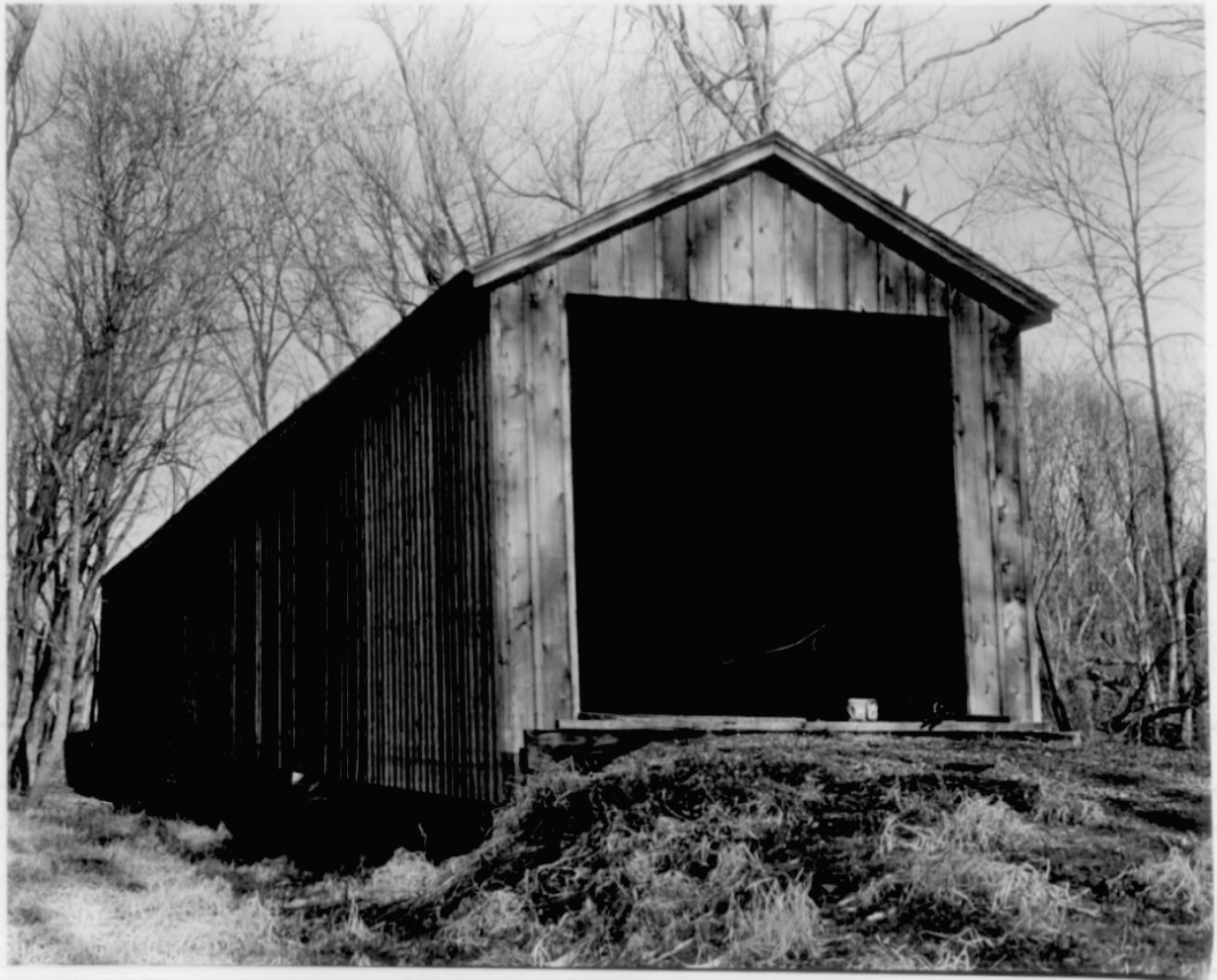
Figure 2-20. Locust Creek Covered Bridge. Photo from NRHP nomination (1970), view to northwest.
