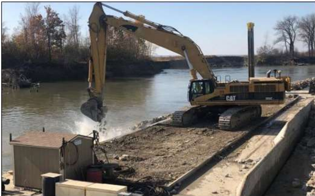
Figure 2-3. Rock being placed to repair/construct a BSNP structure.
