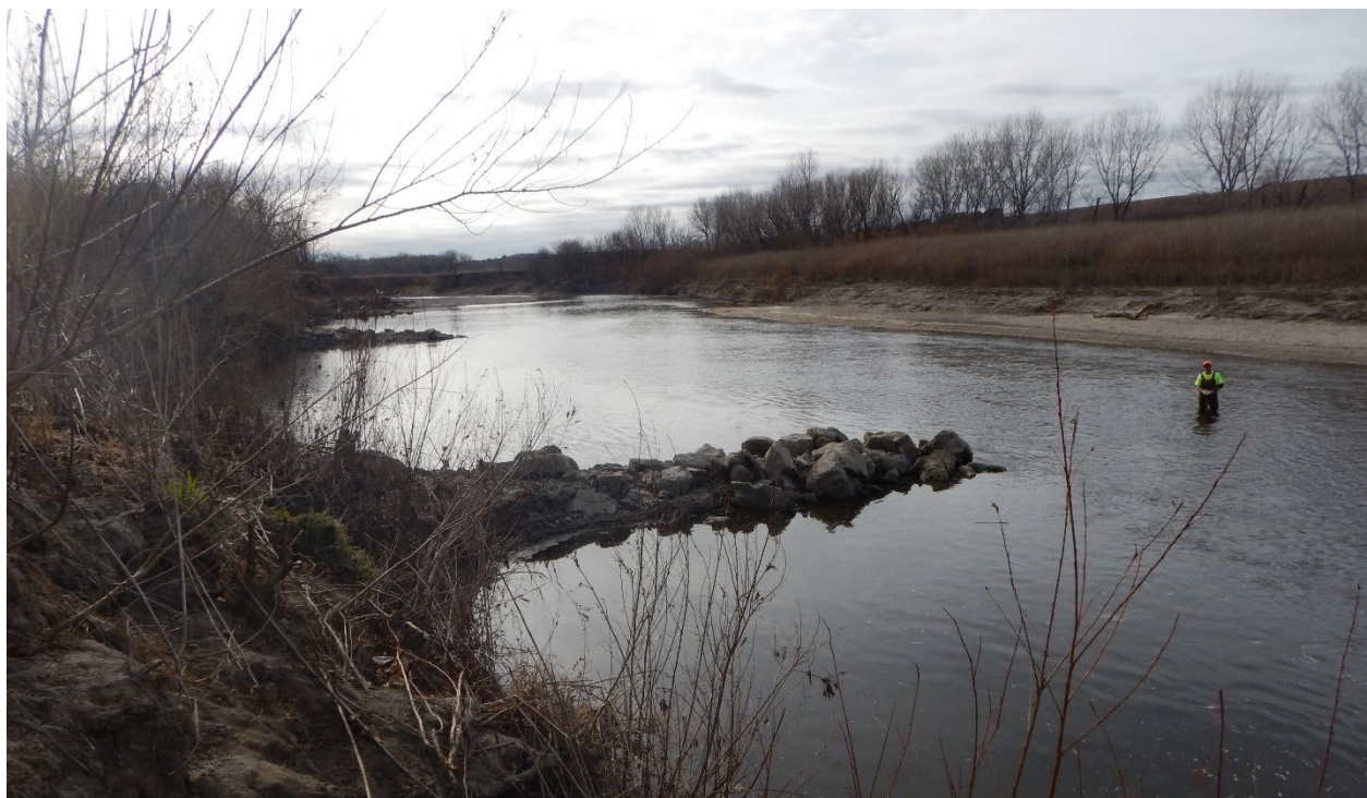
Figure 1: Typical Bank Stabilization Project using Rock Toe and Bendway Weirs (Big Blue River)
