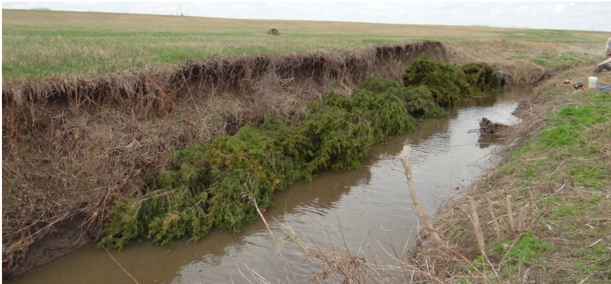
Figure 2: Cedar Tree Revetment on McConnel Creek near Wichita, KS
