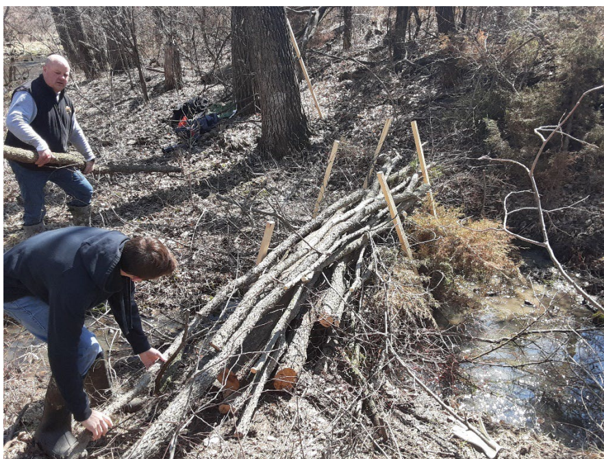
Figure 7. Post-Assisted Log Structure, aka Beaver Dam Analog, Installed by NRCS in Kansas
