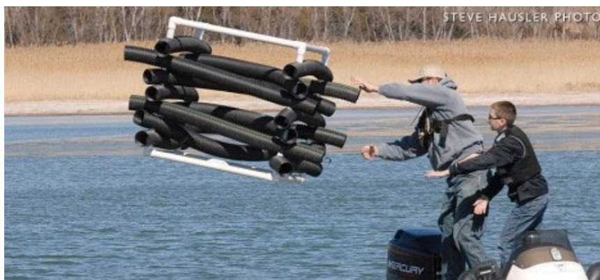
Figure 2. Placement of Georgia Cube for Fish Habitat Improvement
