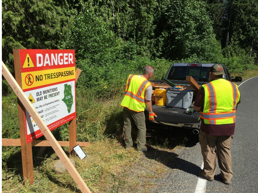
Photo #2: Large Entry Sign (L2) installation along Deer Park Rd
