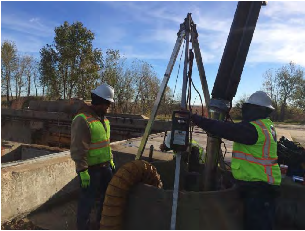
Confined space entry tripod and rescue set up pulley system.
