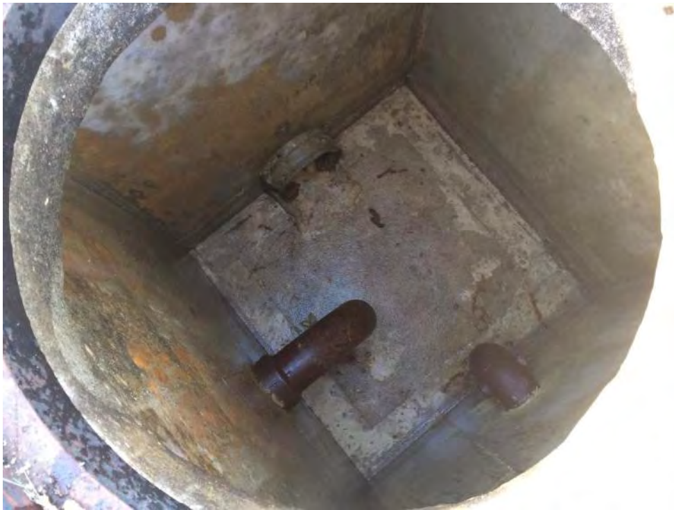
Additional sediment sump pit (cleaned).
