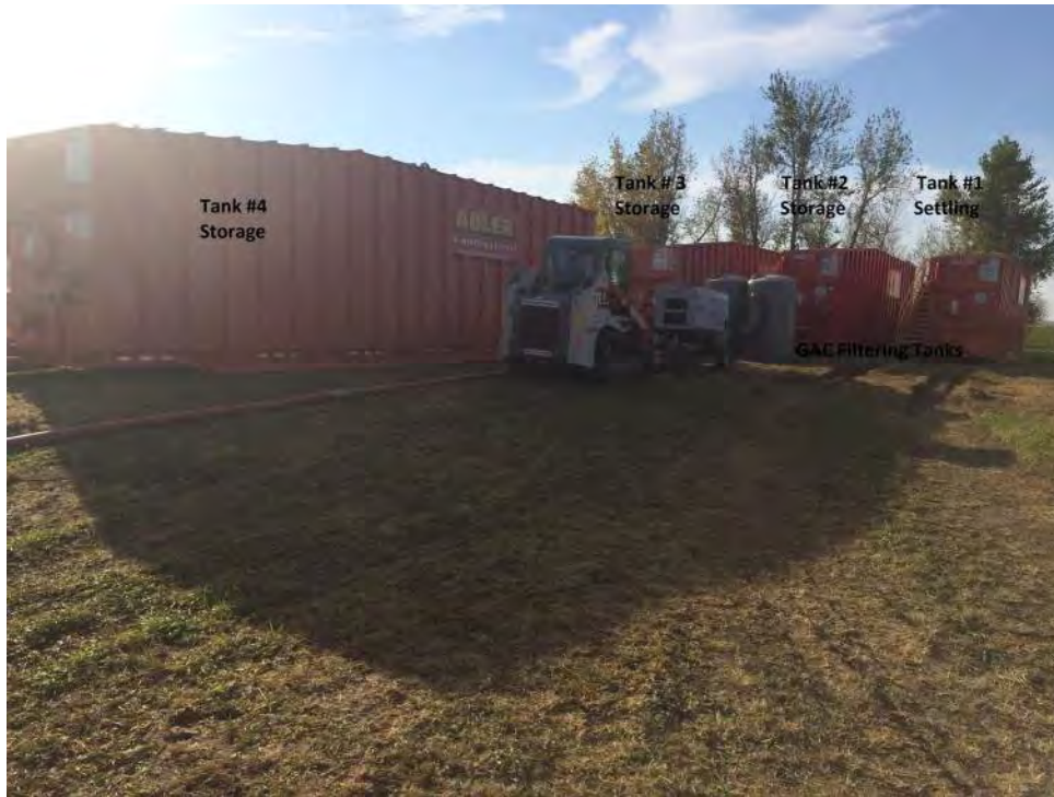
Pump operation set up
