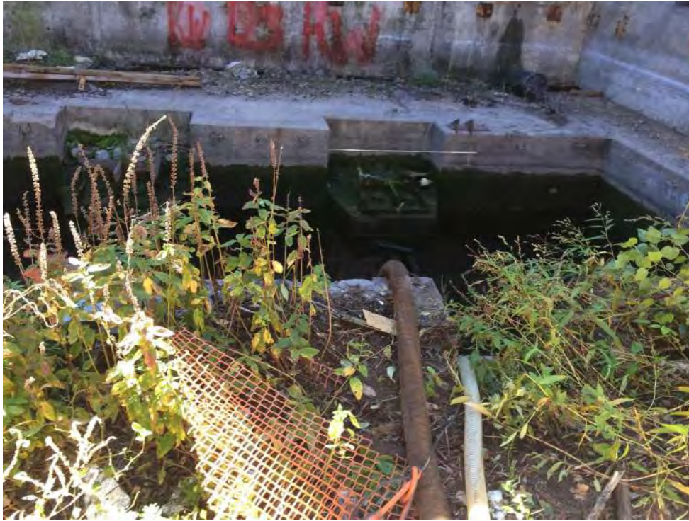
Flame Pit Tunnel.
