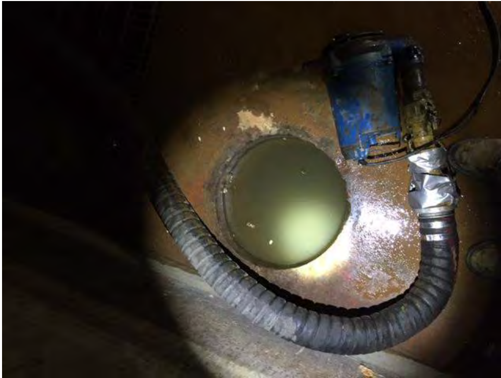
Control Room Sump Pit (before).
