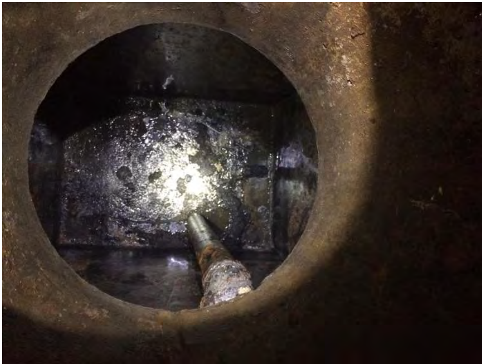
Control Room Sump Pit (After).
