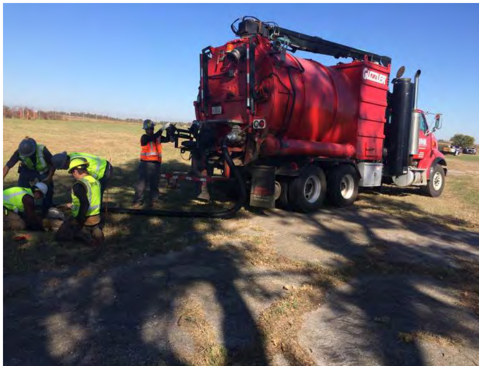
Guzzler Pump Truck in operation (pumping additional sediment sump pit).
