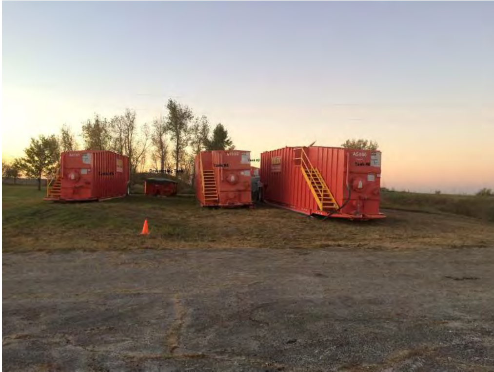
New pump operation set up (added Tank #5 and Tank #6).
