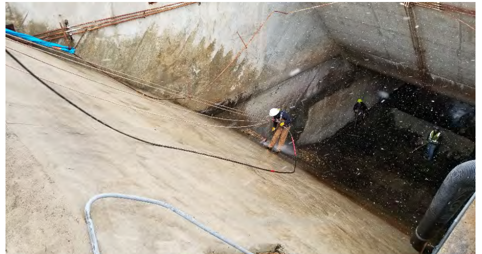
Description: Flame Tunnel Cleaning
