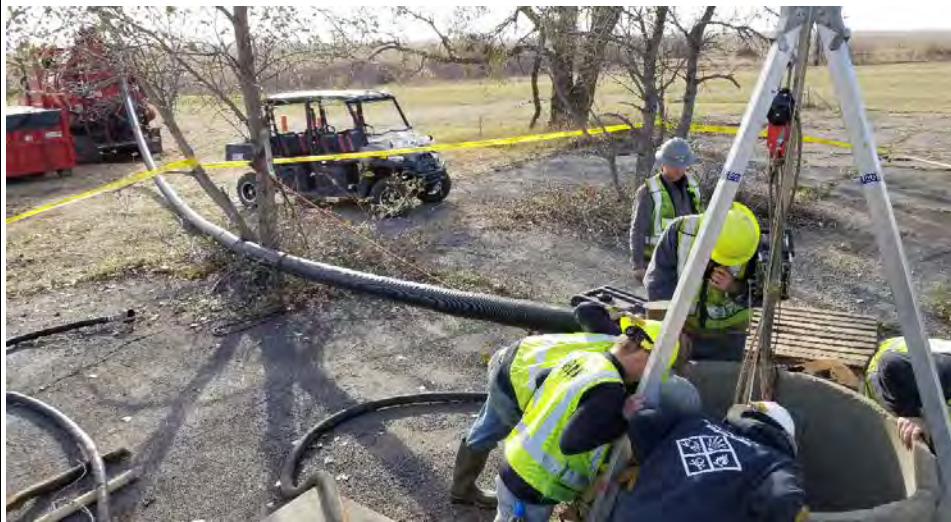
Description: Main Sump Removal
