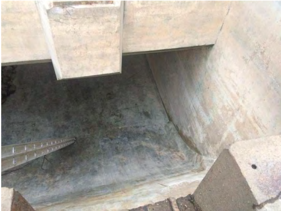
Front side of Flame Pit (cleaned).
