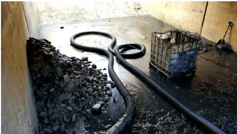
Removing debris from Flame Pit.
