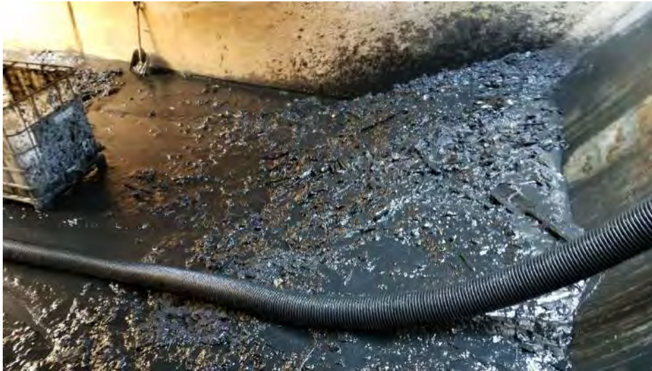
Cleaning back side of Flame Pit.
