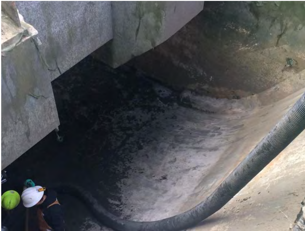
Cleaning Flame Pit.
