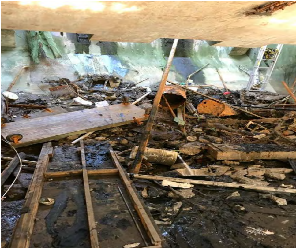
View from inside of Flame pit.
