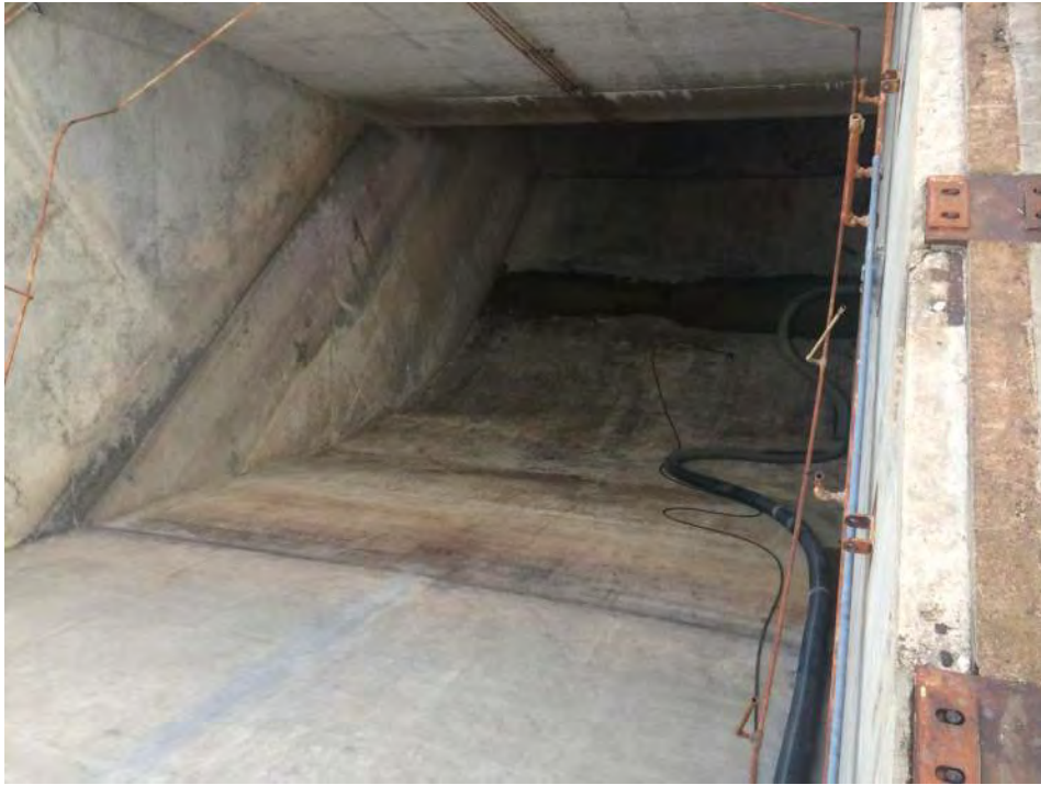
Flame Pit back side (cleaned).
