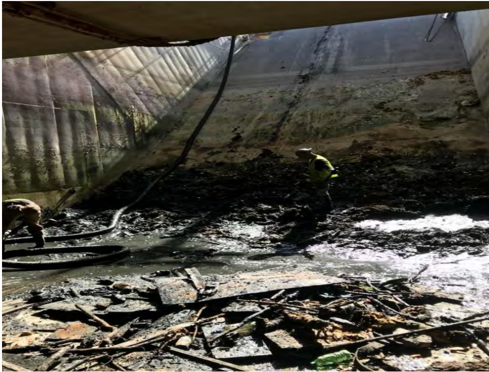
Cleaning Flame Pit.
