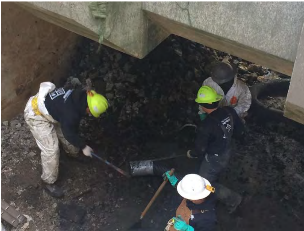
Cleaning and removing debris from Flame Pit.
