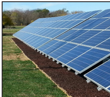
Solar array at Advanced Oxidation Process/Load Line 4 treatment plants
