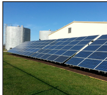
Solar array at Main treatment plant
