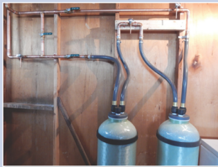
Granular Activated Carbon (GAC) Unit
