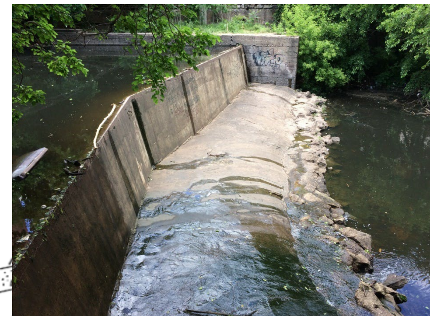
Existing Smokey Hill Dam (Western Star Mill) looking NW
