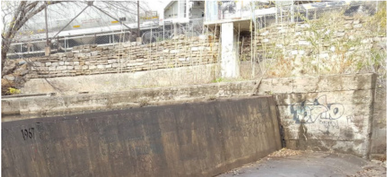
Figure 9. The existing retaining wall at the west abutment of the Western Star Mill Dam. View is to the west, dated Nov 2016.
