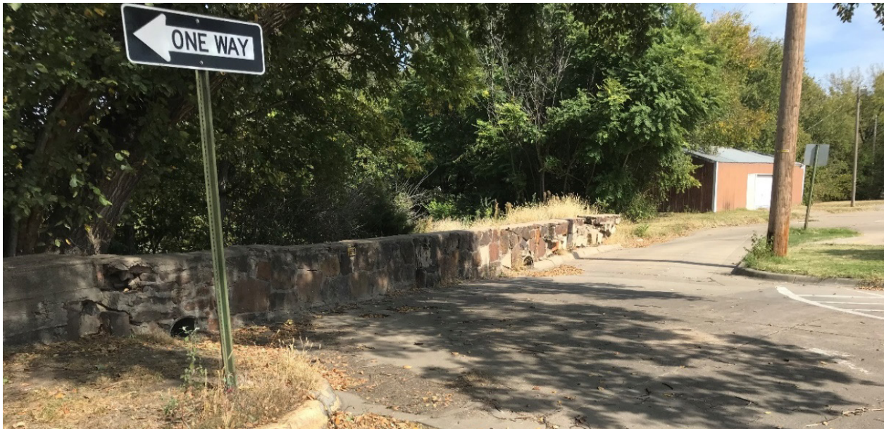
Figure 3. Stone wall at the end of 3rd Street, view is to the northeast.
