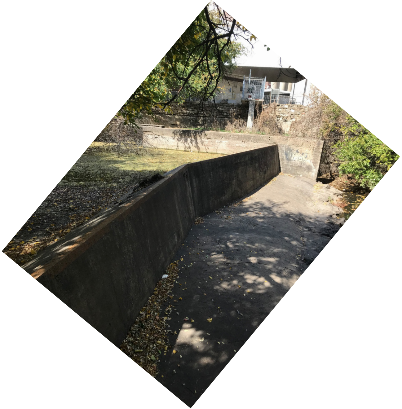
Figure 8. Existing Western Star Mill Dam, looking southwest, dated October 2020.
