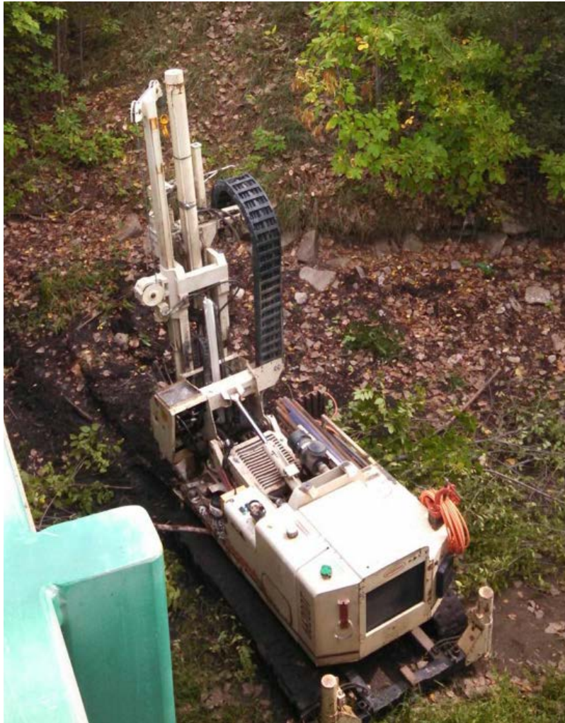
Figure 2 – Geoprobe Track-Mounted Unit at the Bottom of the Channel (Sample ID 12)
