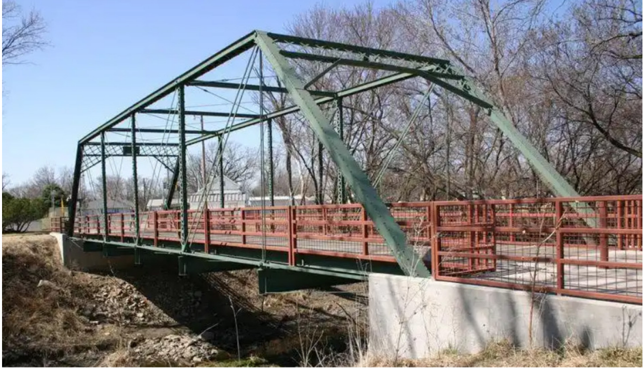
Figure 2. Lakewood Park Bridge.
