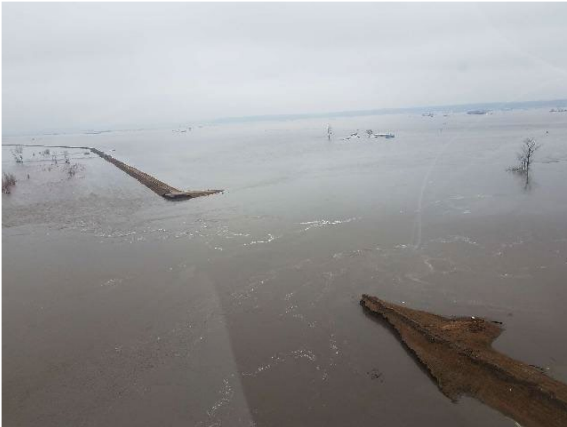
Figure 6: Levee Breach along the Missouri River L-575 Levee System near Hamburg, IA (Photo taken March 2019, USACE Omaha District).
