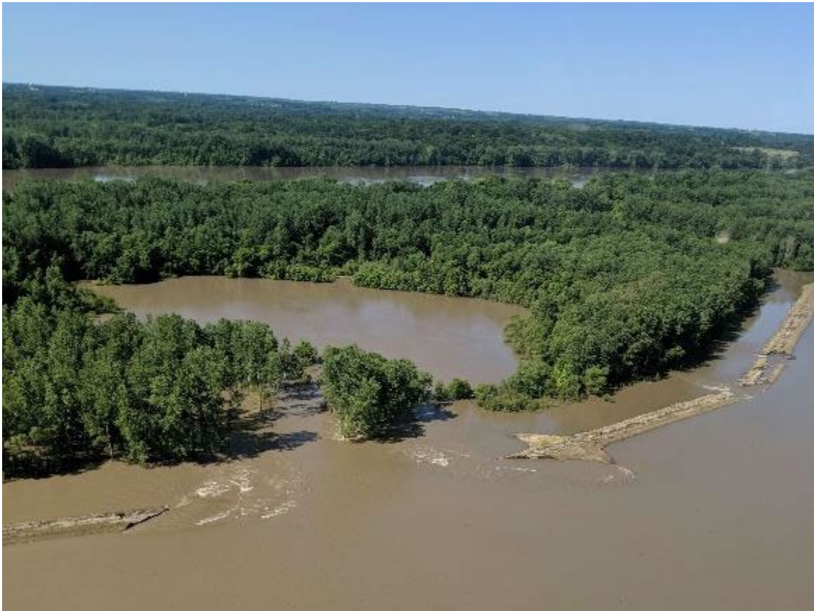
Figure 7: MRLS 246-L Levee System in Chariton County, MO was Breached at Five Locations 2019. (Photo taken June 2019, USACE Kansas City District).
