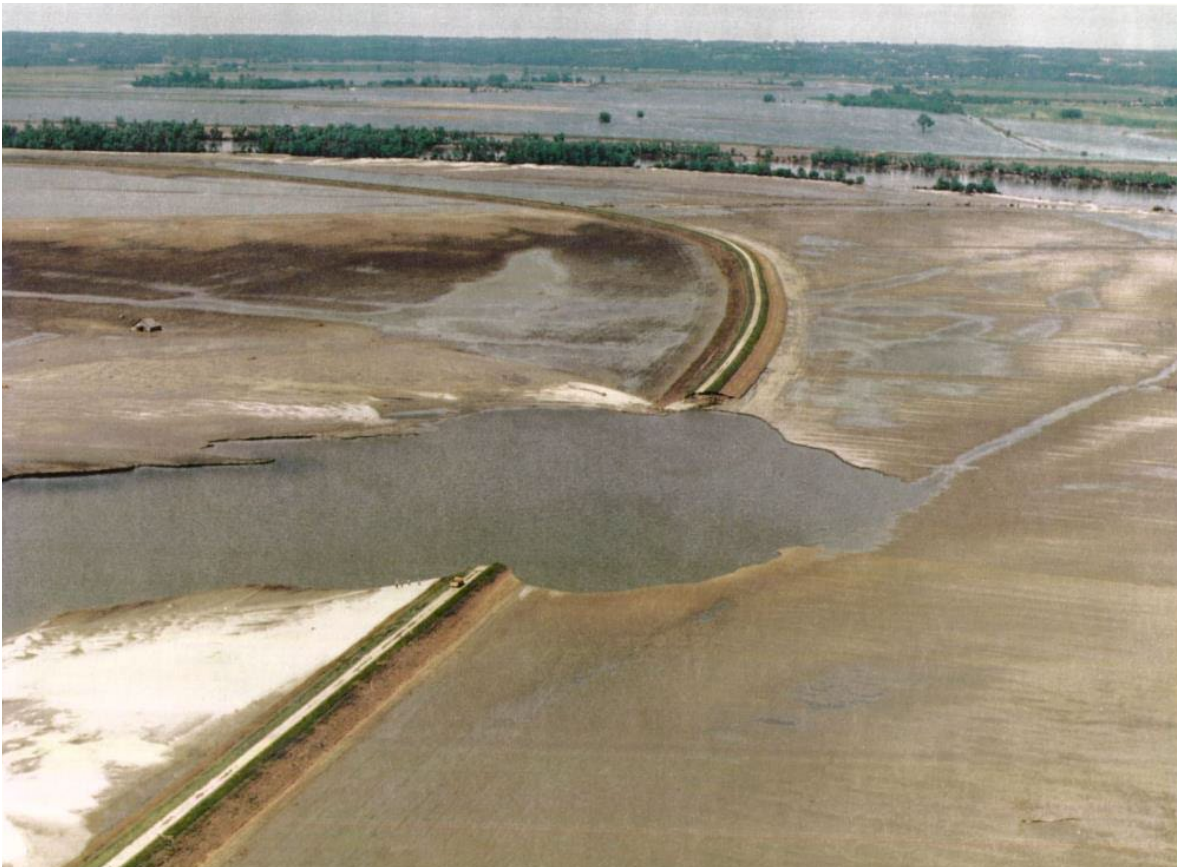
Figure 3: Levee Breach at MRLS 471-460-R, Elwood, KS, 6 August 1993
