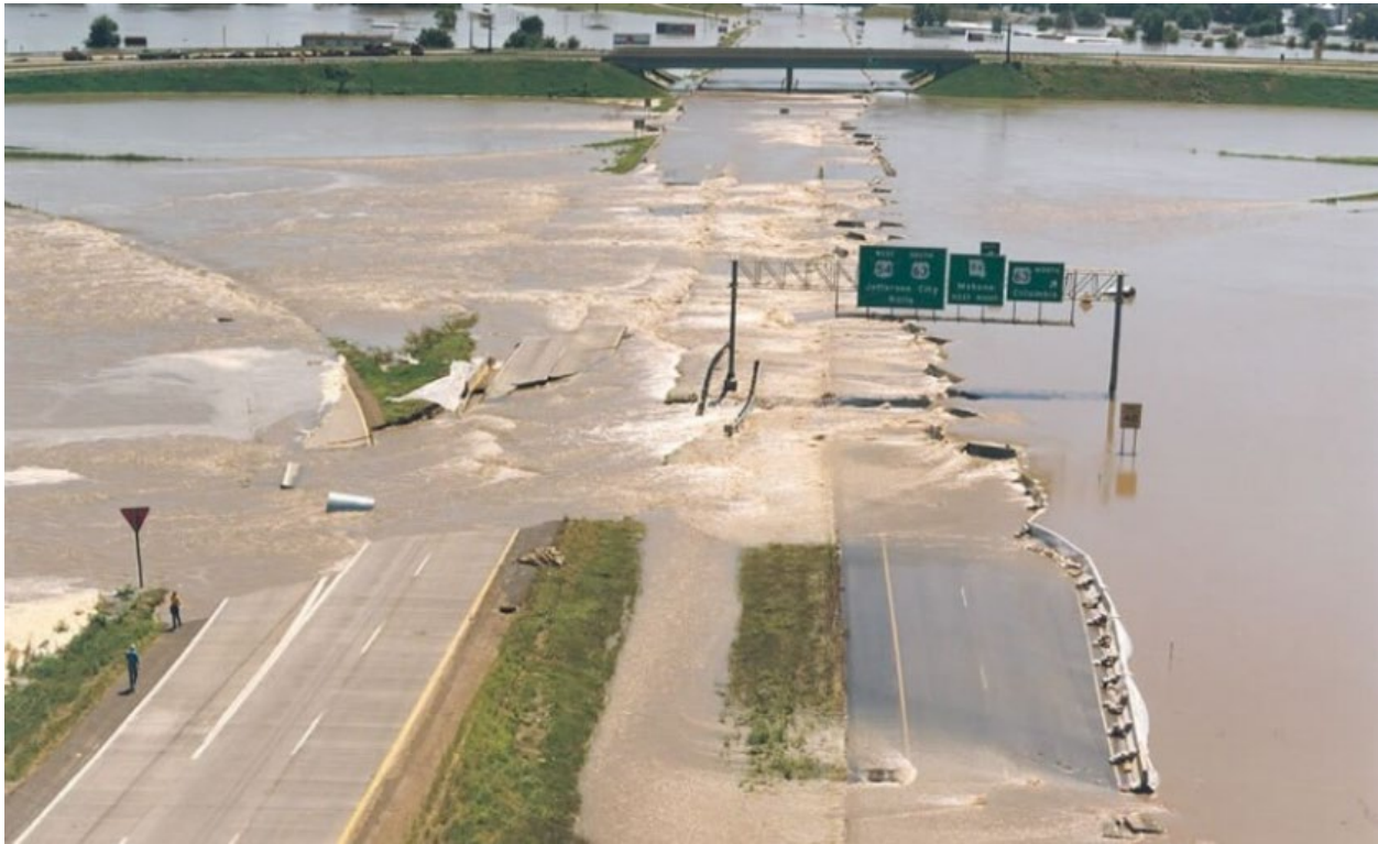
Figure 19: Route 54 Overtopping in 1993
