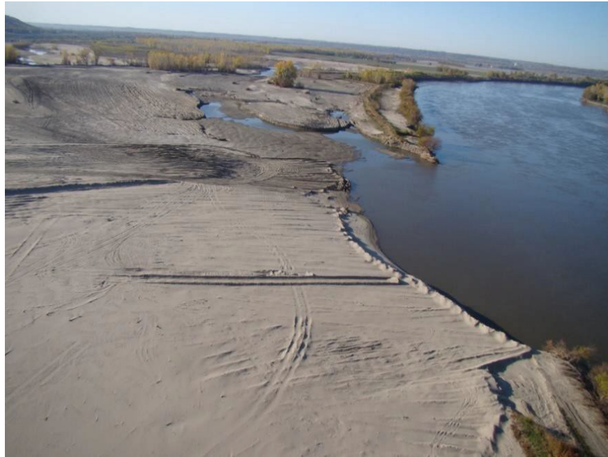
Figure 5: Damaged Levee along the Platte County Drainage District No 1 Section 1 Levee System, Rushville-Sugar Lake Segment near Rushville, MO (Photo taken June 2011, USACE Kansas City District)
